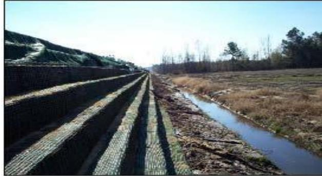
Synteen SR18 is utilized in a variety of soil reinforcement applications such as:
